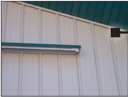
Exterior track cover protects the door system.
