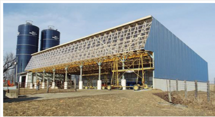
Solar front cattle shed
